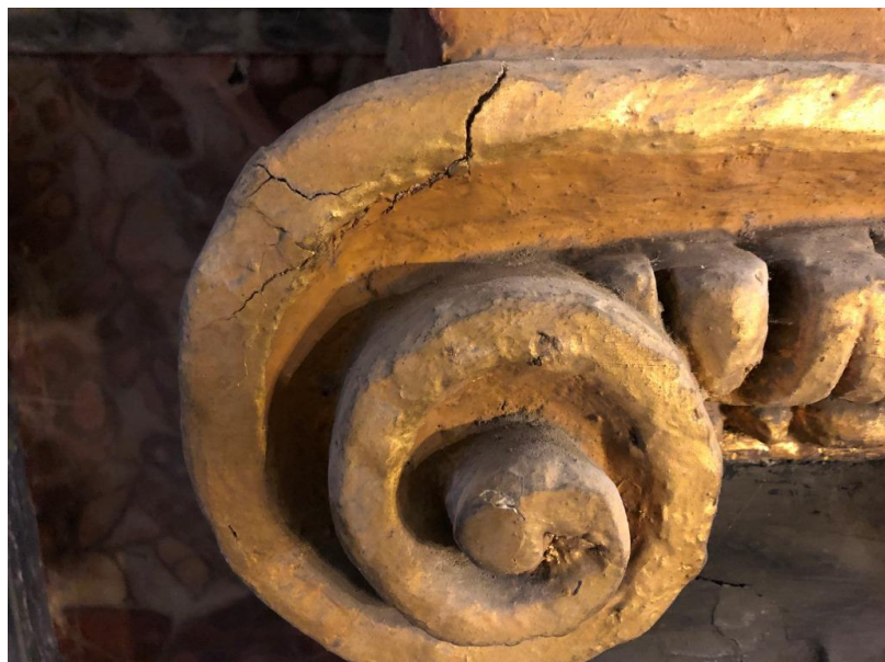
Plate 49: Detail showing the capital above the right-hand column where there is some cracking over hidden iron reinforcement. A metal detector survey of this area gives pretty well constant positive readings – it must be full of iron reinforcement.
