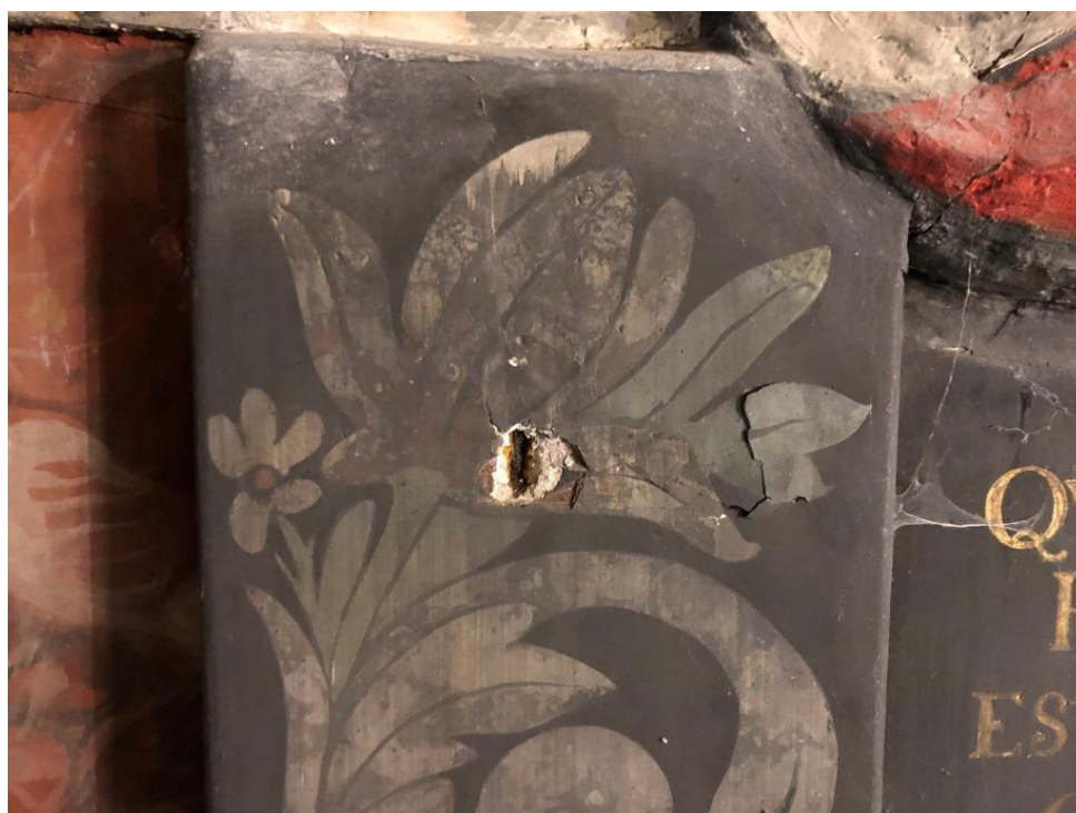
Plate 45: Iron pins – which exactly correspond on the other side – near the top of the frame are also causing disruption including, here, flaking of the plaster surface.
