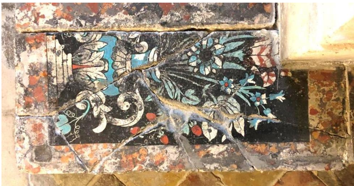
Plate 32: Panel 3, which is badly broken up and has been previously repaired with cement.
