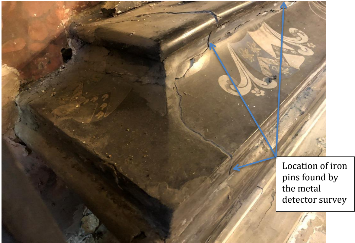
Plate 42: Detail of the upper parts of the sarcophagus, showing cracking and structural disruption associated with the location of ferrous fixings.
