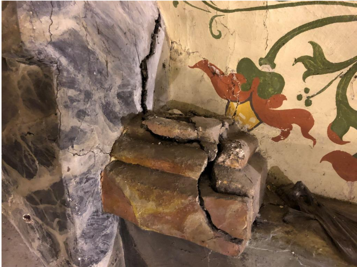
Plate 50: Detail showing the interface of the wall and the monument bust to the right-hand side of the central cartouche. The cracks and disruption is at the join and has caused a fair amount of disruption.
