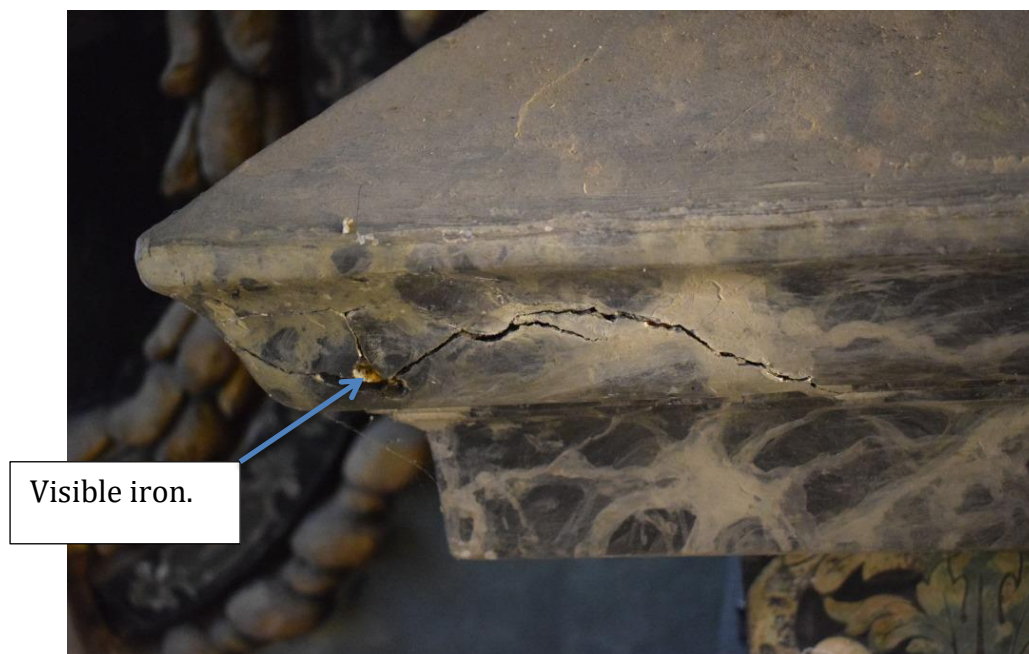
Plate 46: Localised surface disruption and cracking to the cornice where a section of iron reinforcement is corroding.
