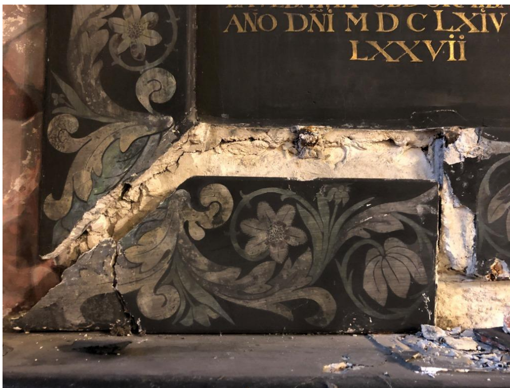
Plate 44: Where the lower parts of the frame have come away the corroding iron cramps, and sectional make-up of the frame, can be clearly seen.
